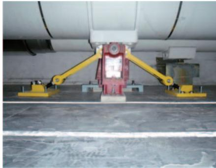
Fig. 6. – (Colour on-line) The reinforcement (yellow parts) on the floor supports of the SSS with vacuum barrier.
